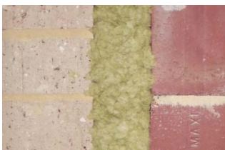
Typical cavity masonry installation detail
